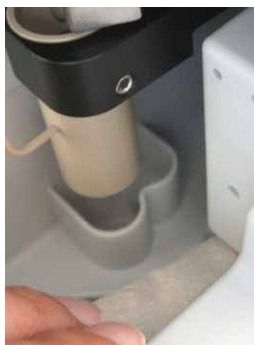
Fig. 39: Drying the leak sensor
